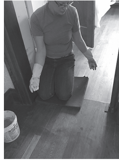
Refinishing the living and dining room floors
