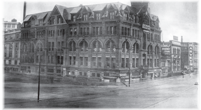
The Kuhns Building at 4th and Main Streets
