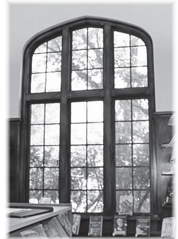
The large windows in the reading rooms unite the library with its setting.
